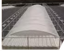
Continuous Vaults and Ridges with Ventilation Systems
